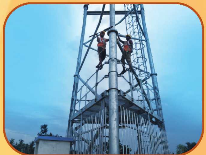
Mobile Towers Maintenance
